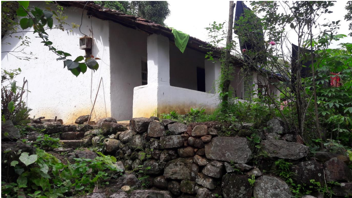
Picture 1: A Deteriorated Govigama house, Teripaha
